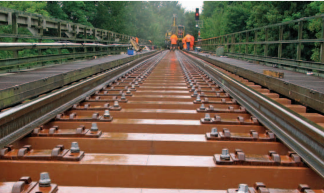
Reinstating the rails following installation of the FFU bearers.
