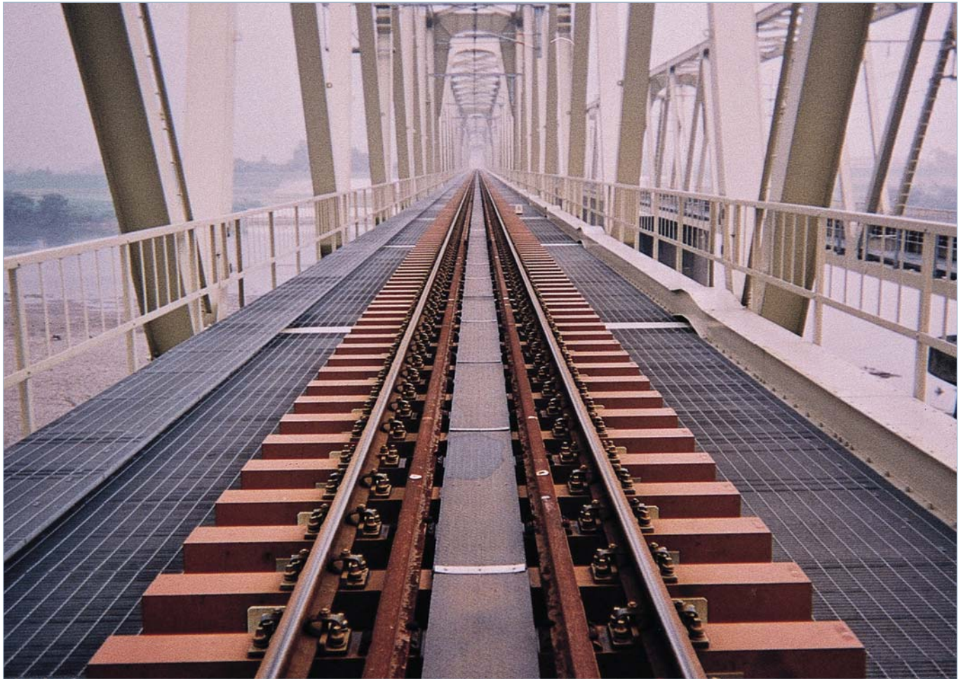
FFU Synthetic Wood on Steel Bridge - Japan - [SEKISUI]
