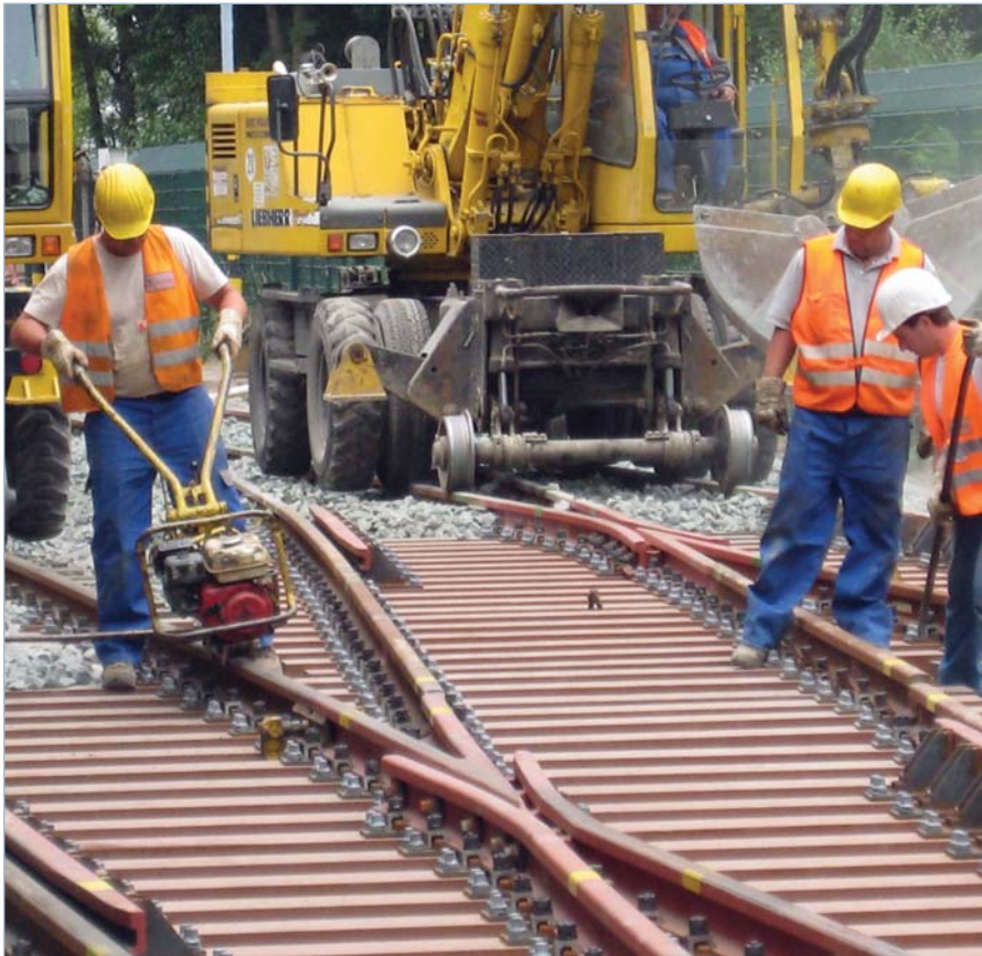
Turnout Installation at Chempark Leverkusen-Germany-[SEKISUI]
