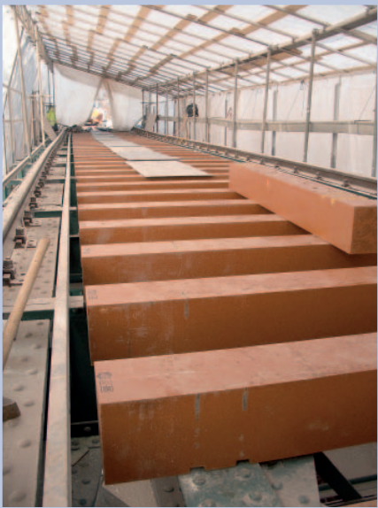
Fig. 4: The ÖBB's Karwendel bridge in Innsbruck (Photo: koocoo consulting)
